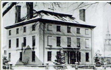
Pre-1881 Stucco House
